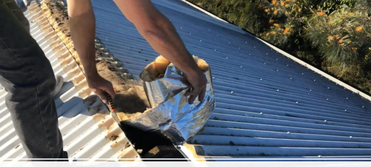
4. Cut back any insulation or anticon to reveal throat gap
