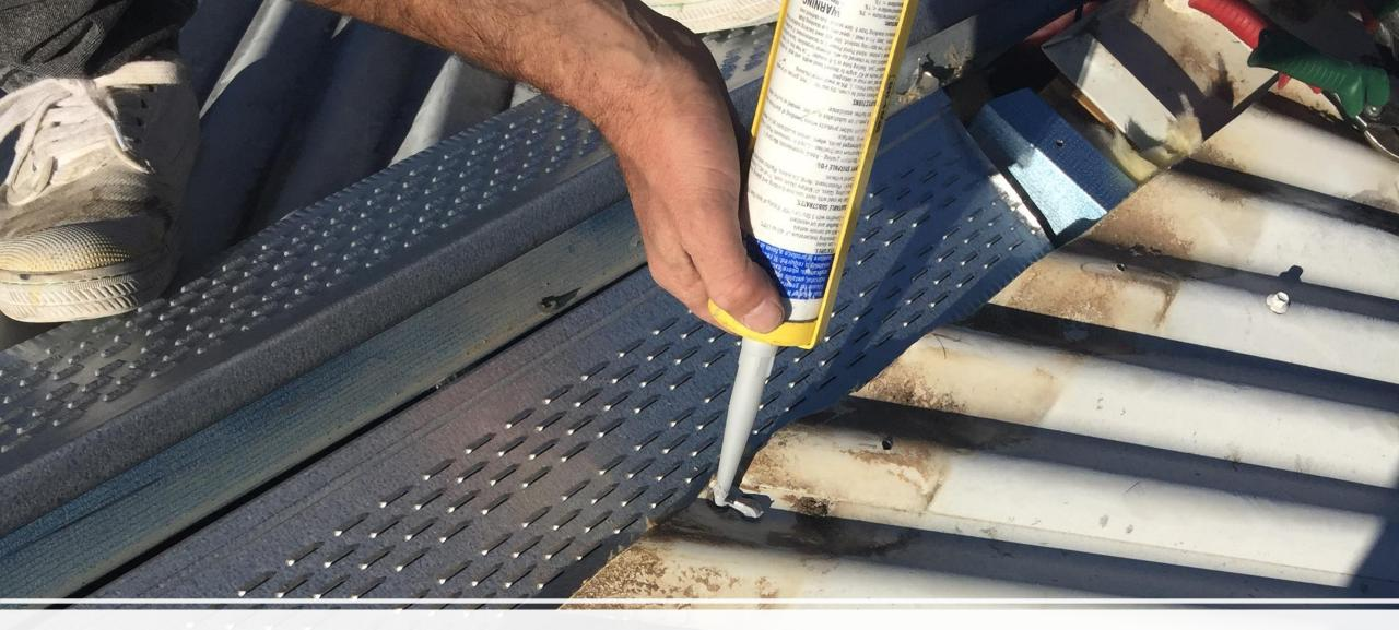
7. Apply silicon to each louvre join – also silicon pre-existing screw holes as you go
