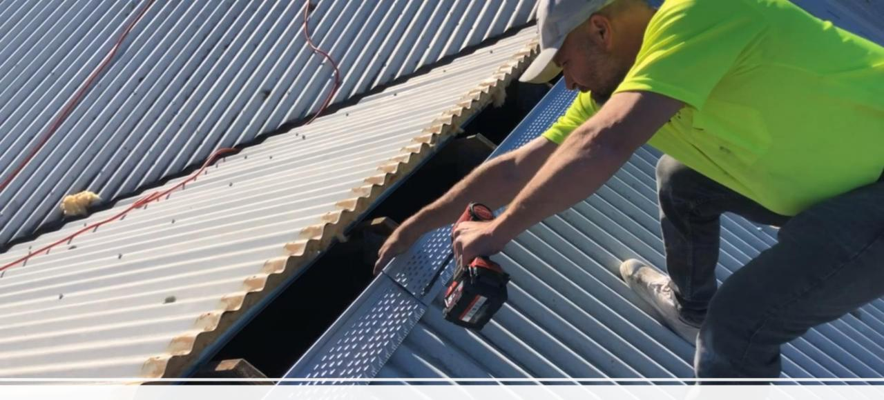
6. Ensure foam is imbedded at least 3mm into roof sheet. This creates a watertight seal
