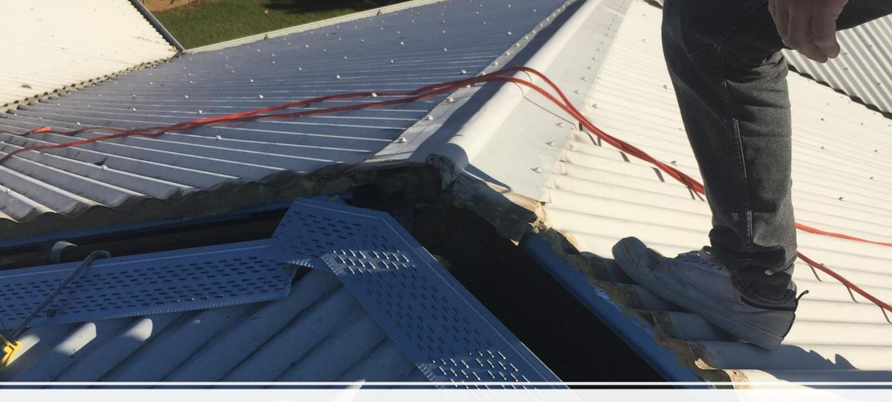
8. Snip hip sections to allow louvre to bend around corners
