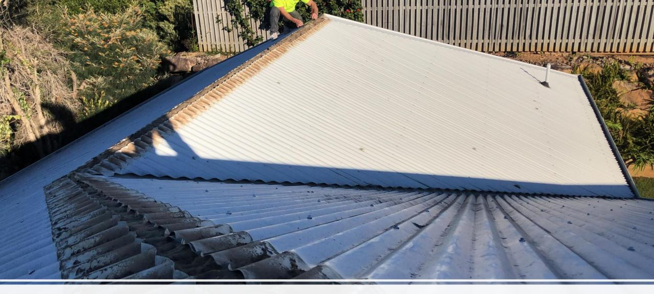
2. Ping a line across the ridge in preparation to cut the sheets back
