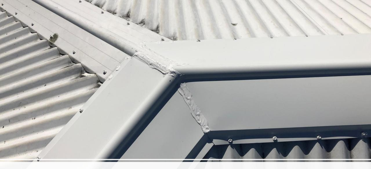
9. Install ridge as usual, molding the new ridge into the existing ridge
